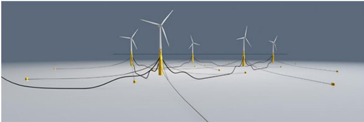
Each anchor resembles an upturned bucket. Water is pumped out creating a vacuum inside, which makes the bucket penetrate down into the seabed. The suction anchors at Hywind are 5 metres in diameter and penetrate 15 meters into the seabed.
