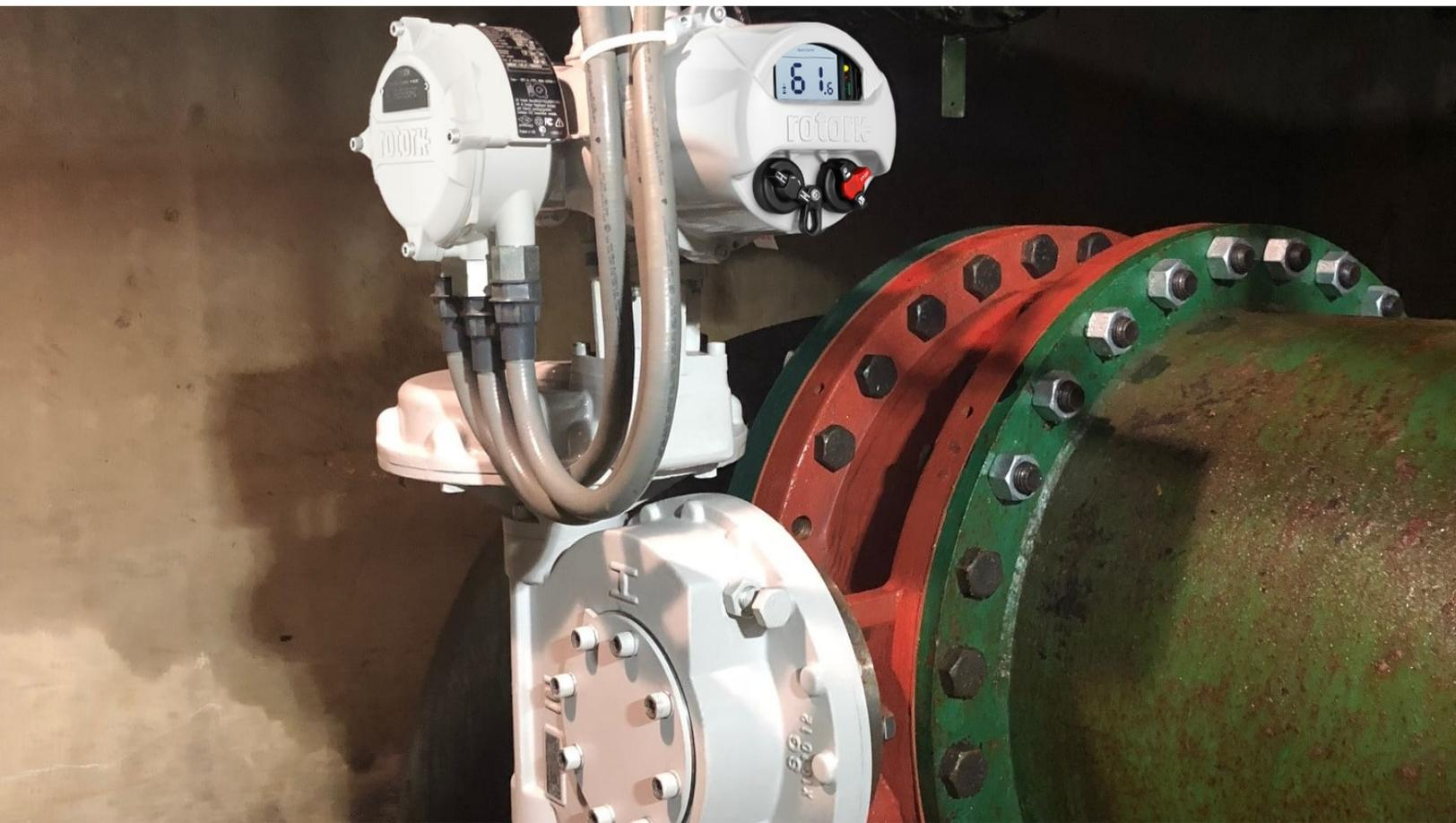
The Rotork IQ electric actuators with IW gearboxes are controlling the inlet and outlet flow of raw water at the Eugene Sawyer Water Filtration Plant sand filter.
